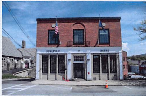
SULLIVAN HOUSE CLAREMONT | 28 beds Recovery Housing (Supportive Housing)
